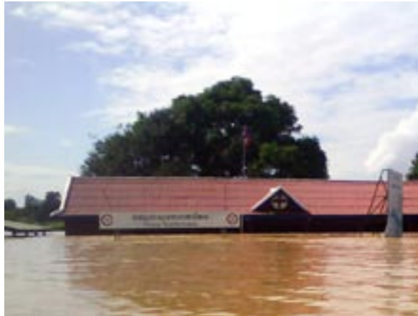
Taveng Health centre under water
