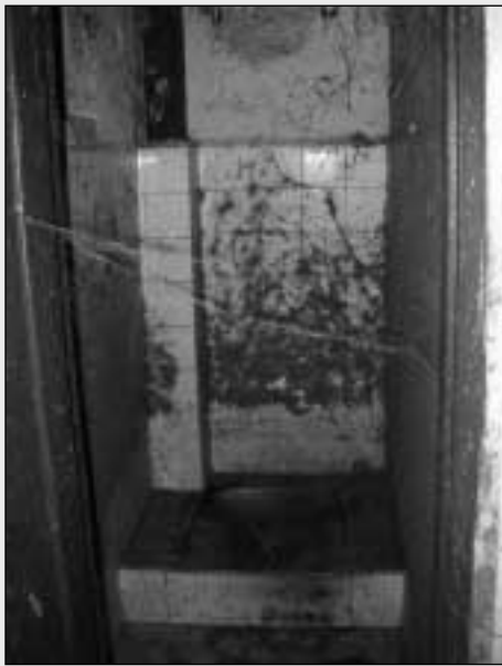
the toilets ...before
